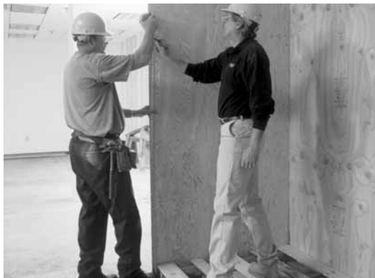
Many crews speed up the stacking by building a simple two-sided, free-standing frame. Note: Frame is not attached to pallet.
